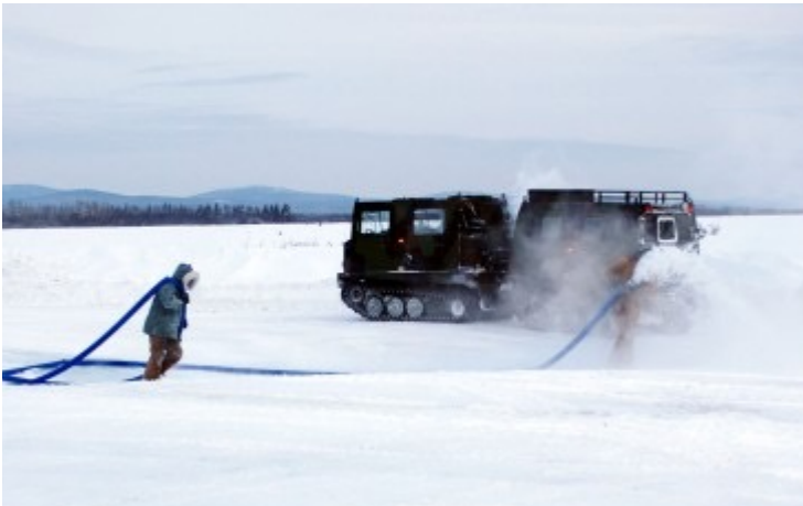
Soldiers reinforcing an ice bridge on the Tanana River, Fort Wainwright, Alaska.
